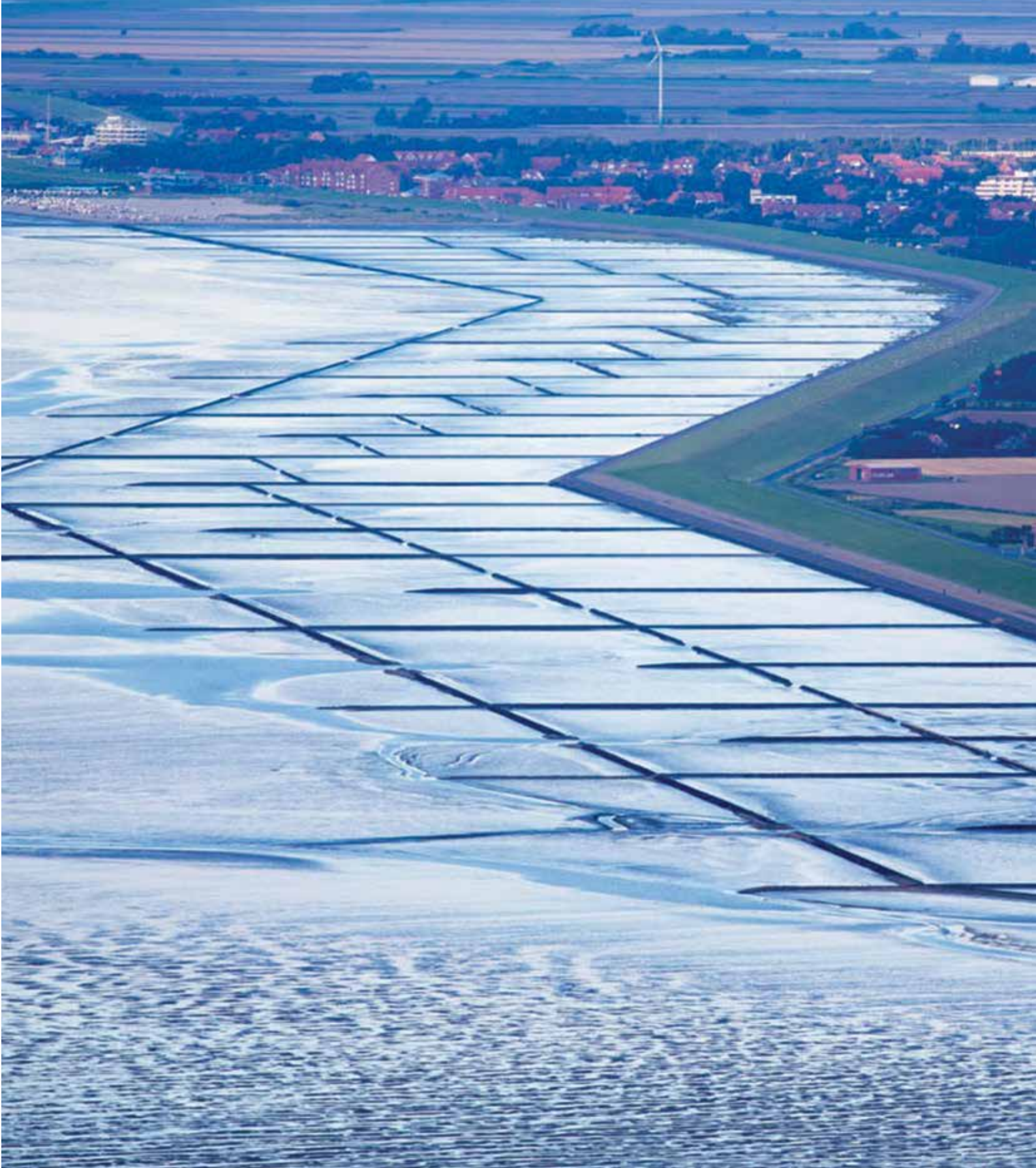
A lattice of jetties in front of levee traps silts to extend the land mass (Norden, Lower Saxony, Germany).
